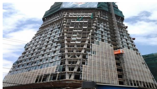
Fig. 12: Britam Towers, Façade construction, Nairobi, Kenya ( Welch, 2018 )
