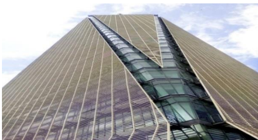
Fig. 7: Britam Towers, exterior with fixed egg-crate solar-shading system design made of Terracotta Ceramic Rods (PamGolding, 2018)
