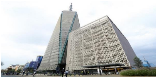
Fig. 10: Britam Towers, exterior with fixed egg-crate solar shading system design made of terracotta ceramic rods ( PamGolding, 2018 )
