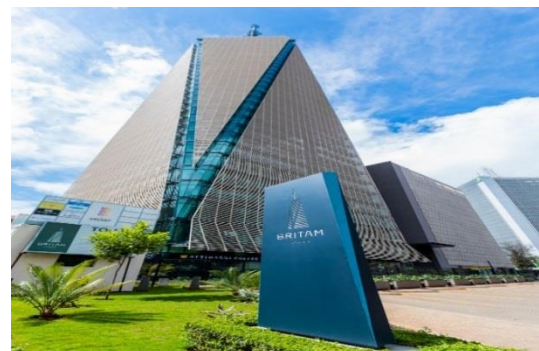
Fig. 9: Britam Towers outside façade, showing solar-shading system and tinted blue glass, Nairobi, Kenya (Welch, 2018)
