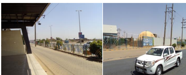
Fig. 7: Difficult access car and pedestrians' access (Burri Park)
