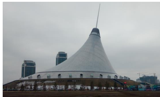
Fig. 20: View of the Khan Shatyr entertainment center (Nurumova, 2017)
