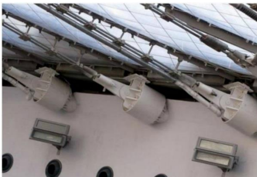
Fig. 22: Cables view (Nurumova, 2017)
